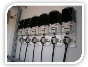
the modules at ground level. To facilitate this safety innovation, these new retractable towers can no longer use the large and bulky copper wire bundles of 'yester-year'. Instead, they require small gauge wire loops, which expand and contract as the PV array is raised and lowered. Morningstar's TriStar MPPT Controllers help to efficiently enable these systems' to work without voltage losses, using a more cost-effective lower gauge wiring solution.
