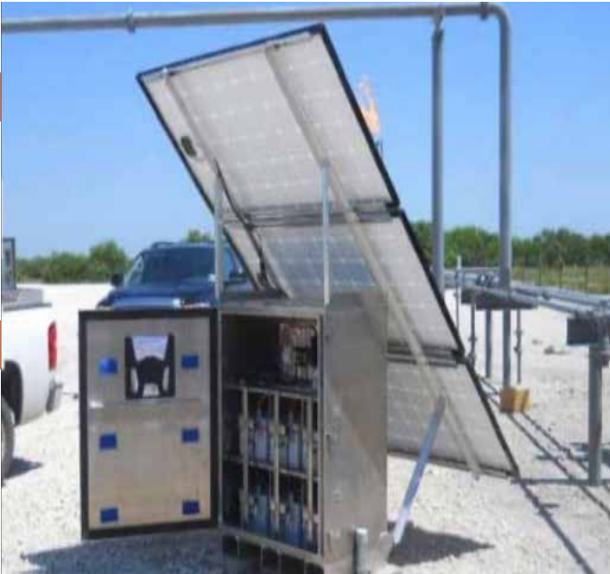
SunSavers in remote powering system by Deka Solar and Ameresco, Eagle Ford Shale site in Texas
