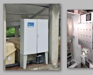
Designed for a wide range of standard telecom BTS and microwave relay sites, the Apollo Solar Series supports pure solar or hybrid (grid and/or genset) site powering scenarios. The typical installation has 3-20kW PV per site; systems also often serve "multi tenant" sites (multiple MNO or Virtual MNOs, for example).
