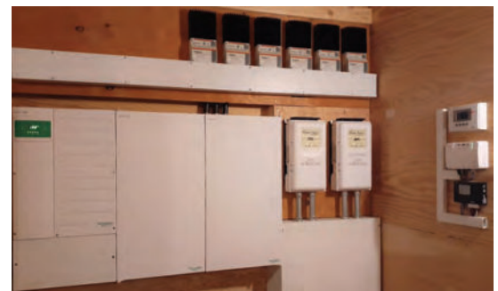
Viridian's micro-hydro load diversion or "dump load" arrangement, using six Morningstar TS-60A controllers
