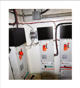
Telecom station with 600V charge controllers at McEvoy Lake, Canada
